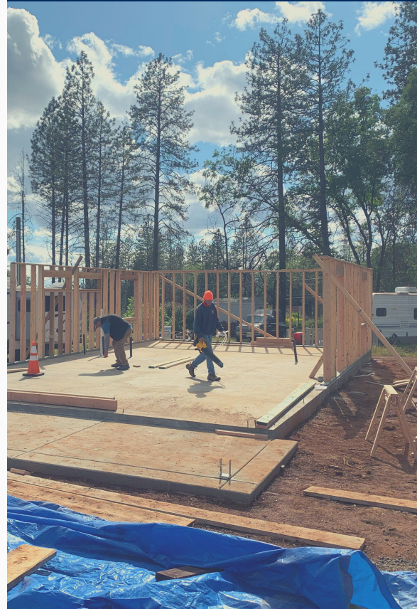
A team of volunteers frames our first home rebuild in Paradise
