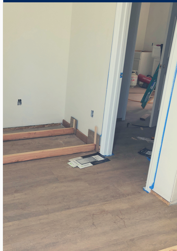
Center photo: Step Foundation being framed.
