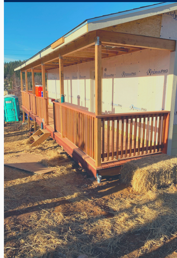
An HCRN home being rebuilt in Northern California
